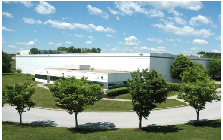
Exterior of 6695 Business Pkwy in Elkridge, MD
